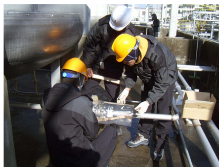
Sealing of a fugitive source
