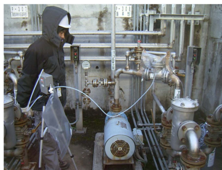
Sampling of the fugitive emission gas
