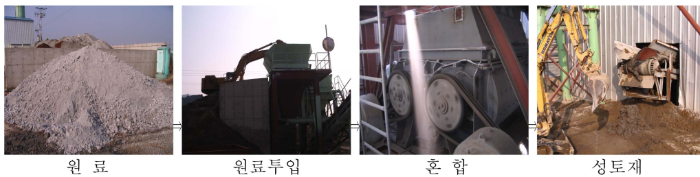
Fig. 4. Manufacturing process of fill material for polysilicon sludge.
